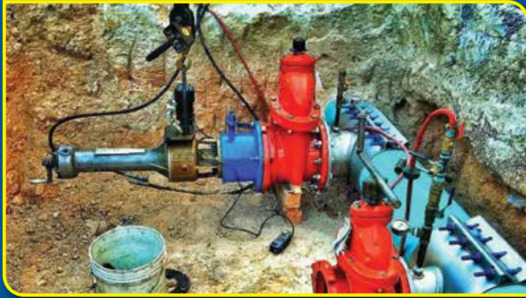
10" WET TAP ON C-900 PVC PIPE
