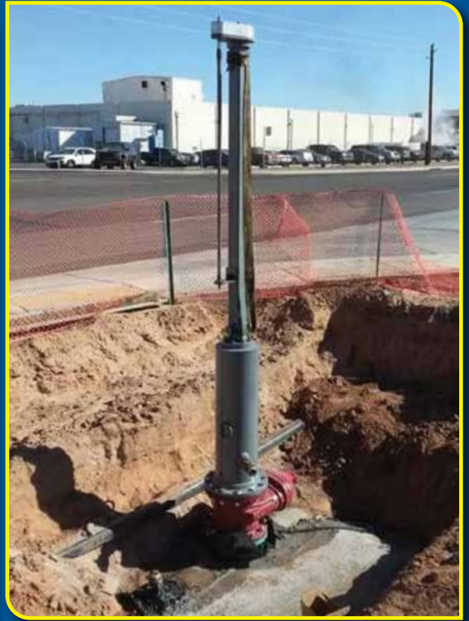
SINGLE 16" x 12" LINE STOP ON AC PIPE
