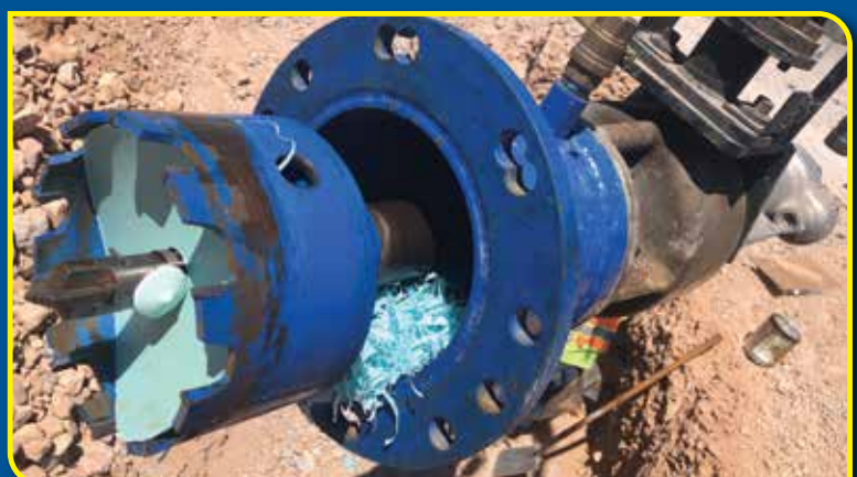
10" HOT TAP ON C-900 PVC PIPE
