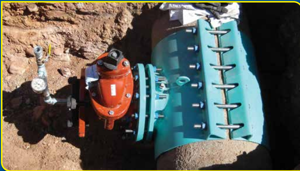
HOT TAP SADDLE FOR CONCRETE CYLINDER PIPE
