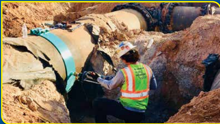
1" SERVICE TAP ON 24" AC PIPE
