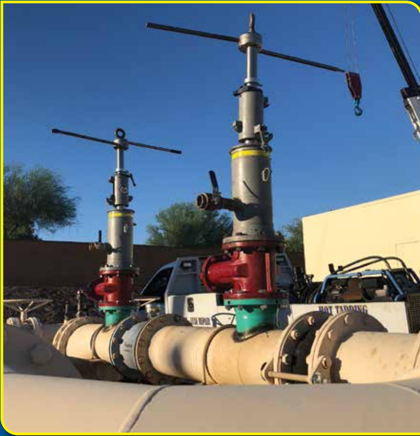
DUAL 12" x 8" LINE STOPS ON MORTAR LINED STEEL PIPE
