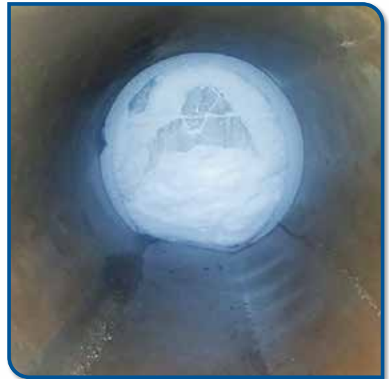
12" PIPE FREEZE ISOLATION PLUG
