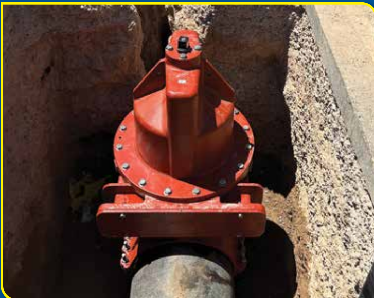
24" VALVE INSERTION ON DUCTILE IRON PIPE
