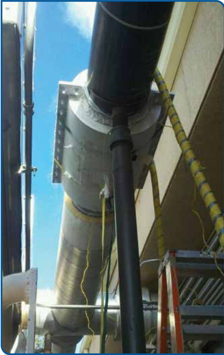
12" PIPE FREEZE ON CARBON STEEL PIPE
