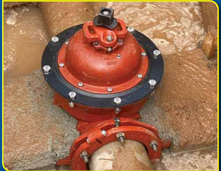
6" VALVE INSERTION ON AC PIPE
