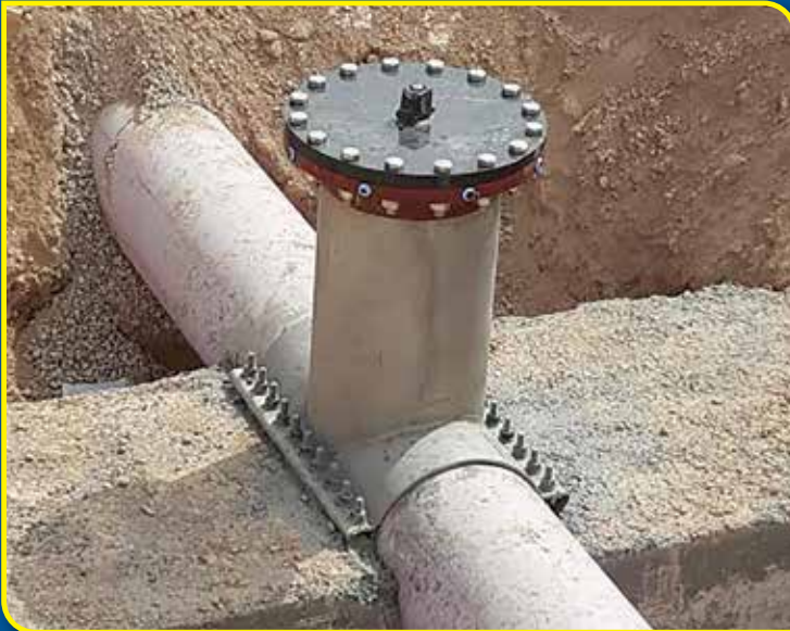
16" VALVE INSERTION ON PVC PIPE
