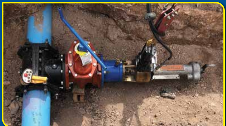
8" WET TAP ON 8" C-900 PVC PIPE
