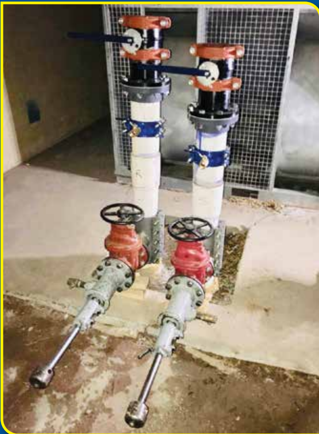
DUAL 6" x 4" LINE STOPS ON IPS PVC PIPE
